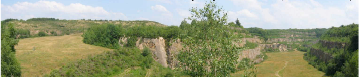
Mill tailings storage site after rehabilitation (MCO 68 - 105, Bellezane)
